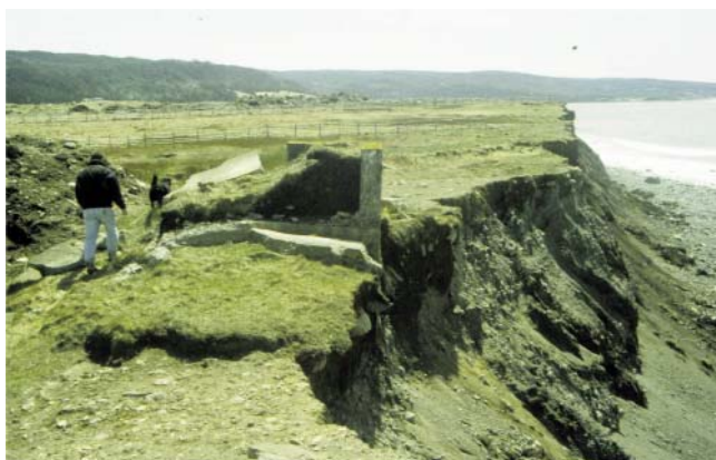
Plate 1. Coastal erosion at Point Verde, Placentia Bay, showing the same structure in 1999 (left) and 2005 (right). Parts of this coastline are eroding at > 50 cm per year, although the average for non-rock cliffs on the Avalon Peninsula is ~20 cm per year.
